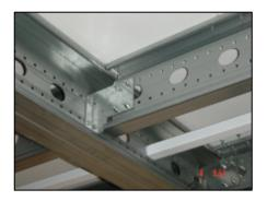
Secondary beams with length > 4000mm have to be fastened with 4 bolts per transverse plate, beams with length <4000mm can be fastened with 2 bolts per transverse plate!
